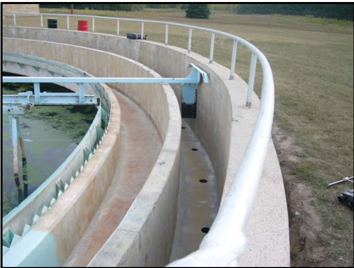
Clarifier Trough Before Polyurea Coating
