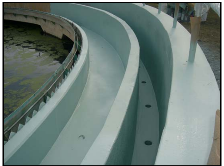
Clarifier Trough After Polyurea Coating
